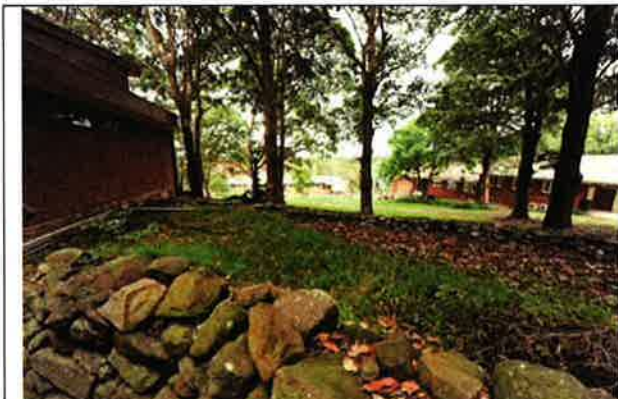
Fig. 86 This image shows how the insertion of the auditorium (at left) cut off the existing dry stone wall. Image by PD, 2010
