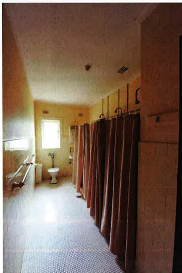
Fig. 51 Bathroom to rear service wing (note: not affected by proposed works)
