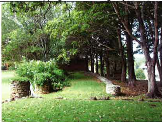
Fig. 89 These 'roundels' have been better maintained, although concrete now holds them together, instead of skilled stone placement. Image MWA 2010
