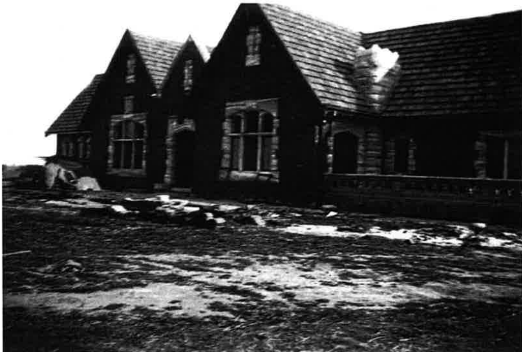
Fig. 4 Gleniffer Brae, east (entry) elevation, 1938, under construction with chimneys and terraces incomplete. Wollongong City Library Illawarra Images, Image No. P18/P18449.
