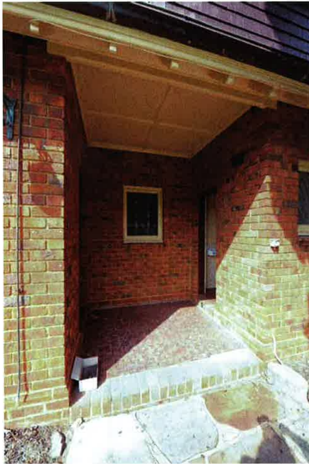
Fig. 48 Rear porch, west elevation, service wing. Proposed works involve alterations to this area for link to proposed pavilion.
