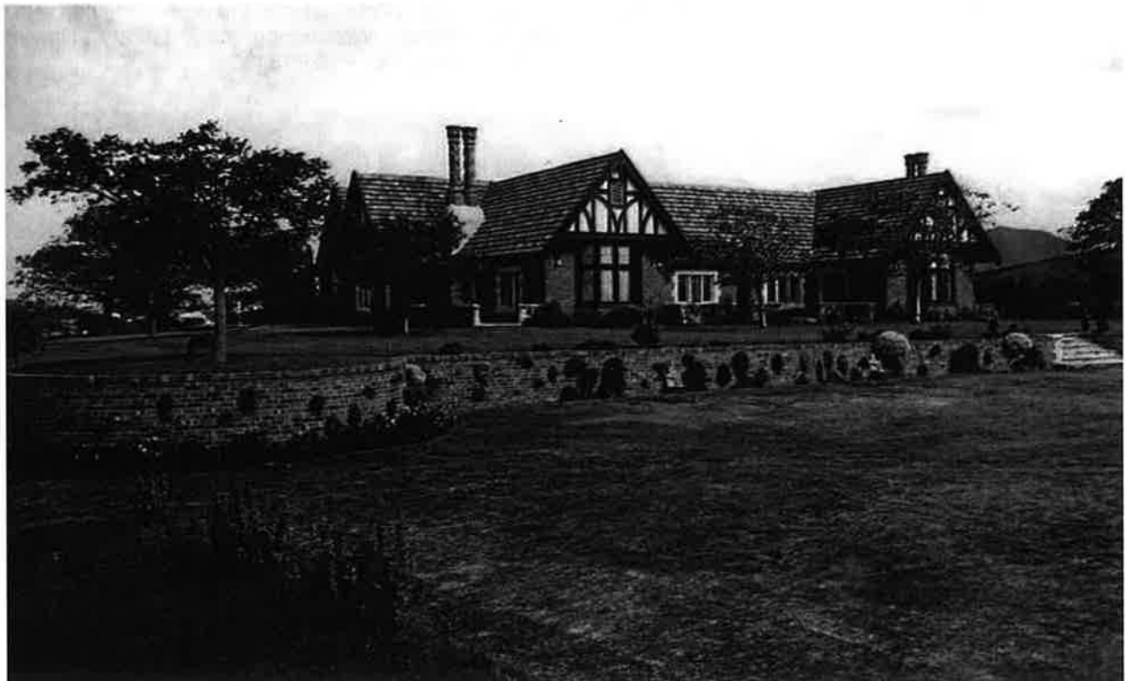
Fig. 5 Gleniffer Brae, north elevation, with roundel of brick retaining wall at left. c. 1940s. Wollongong City Library Image No. P18/P18431.
