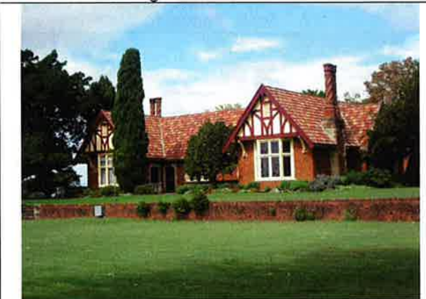
Fig. 26 View of the northern terrace and house. MWA April 2010
