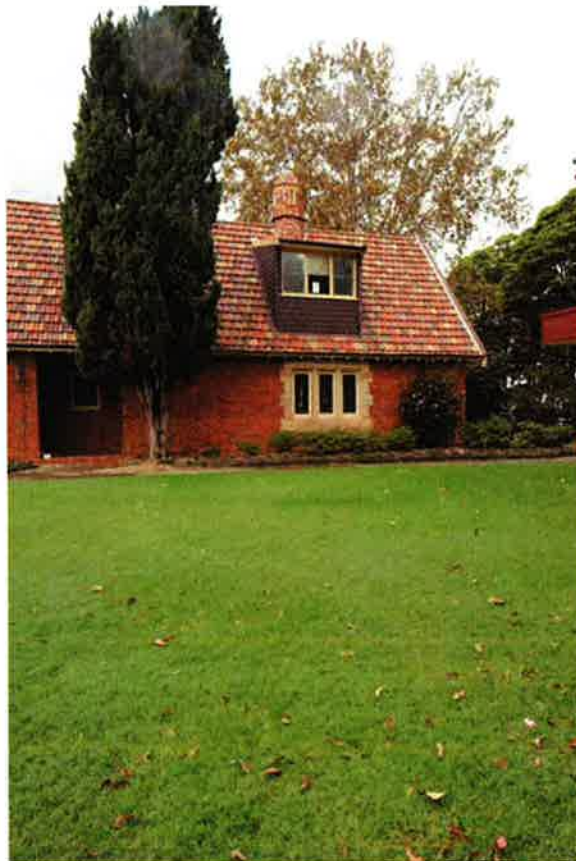
Fig. 45 West elevation of garage (proposed function kitchen). Lawn area in foreground is part of the proposed pavilion location – eave of existing auditorium just visible on right.
