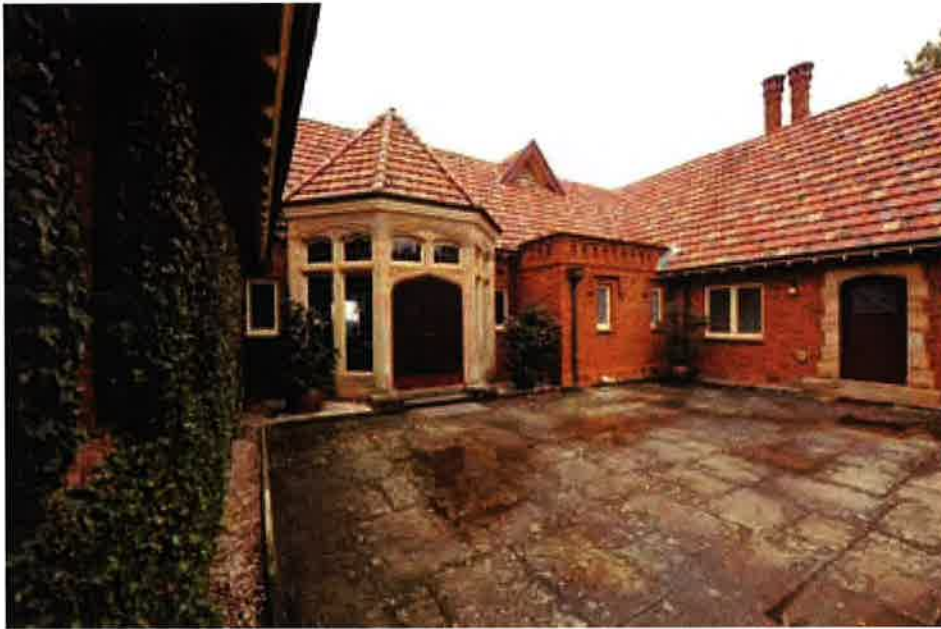
Fig. 40 Rear (west) courtyard of Gleniffer Brae manor house, showing bay window and part of north elevation of rear service wing.
