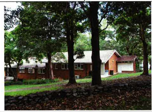
Fig. 25 The school buildings along Robson Road, in the S-W corner, with dry stone walls in foreground.
