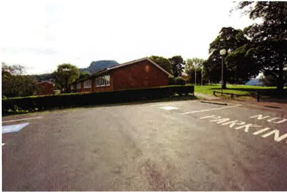
Fig. 63 Anglican school buildings from existing carpark (Mt Keira in background)
