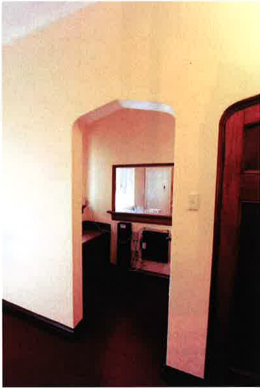
Fig. 52 Former telephone room. Note this is the proposed location for a new disabled toilet and is now rated as low significance
