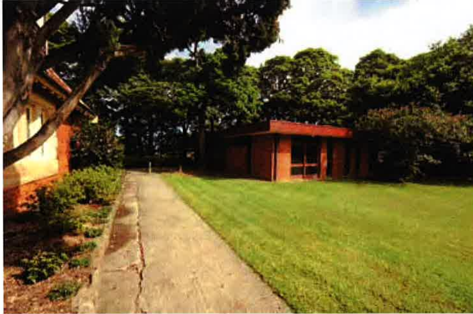
Fig. 59 View of auditorium from north
