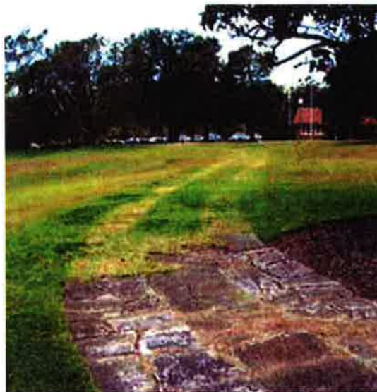
Fig. 81 The foregrounds of this image shows the present condition of the original driveway, the spaces in between having been incorrectly infilled with concrete. The remainder of the return loop is now covered by grass, and it is desired that it be restored to its original state. Image by David Beaver LMP 2007
