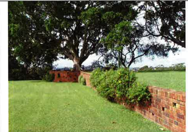
Fig. 27 Detail of the brick retaining wall, with the Sorensen signature 'drum' at the far end.
