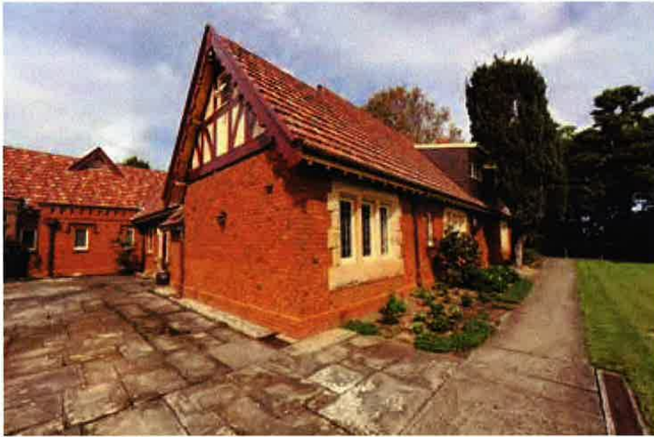
Fig.42 Rear (west) courtyard of Gleniffer Brae manor house and service wing (north and west elevations). Location of proposed pavilion would be on the right.
